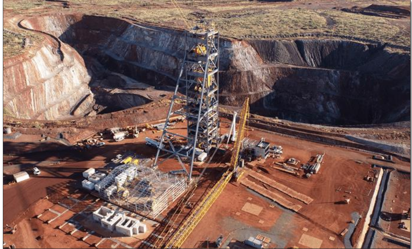
TE2 Headframe – Newmont's Tanami Gold Operations
